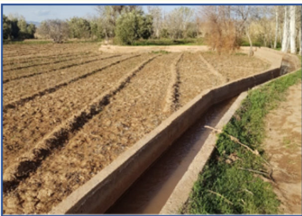
Photo 1: Water diversion of waterways.
