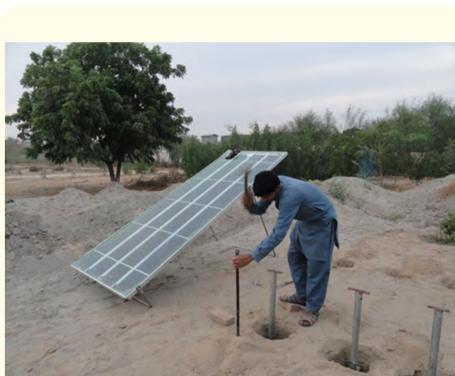
Figure 1: Alignment of poles for solar desalination mounted on pole.
