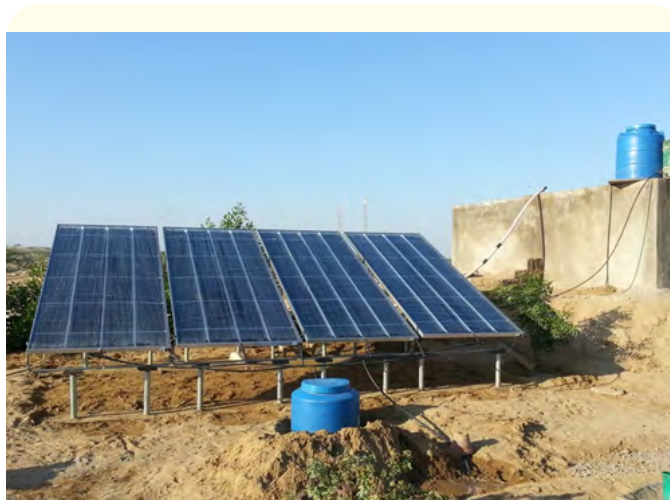
Figure 5: Four units of solar desalination system installed at Gadani, Hub, Balochistan.
