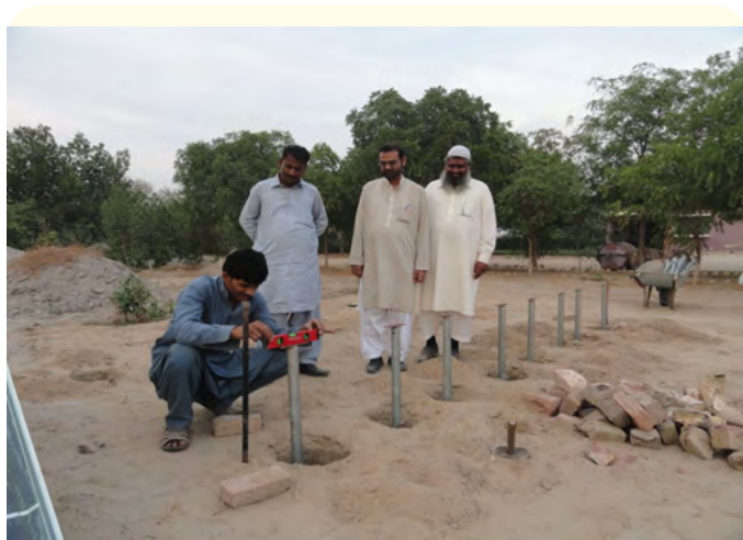
Figure 2: Zero level of poles installation for desalination mounted on pole.
