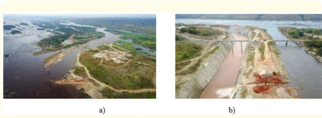
**Figure 3:** Figure 3a) offers a view of the Congo River in the Inga site. Figure 3b) offers a view from the Congo river of two parallel water intakes feeding the Inga I and II power plants during construction and after the commissioning of the second intake of the Inga feeder channel in 2018, (Artélia 2018 Pictures).
