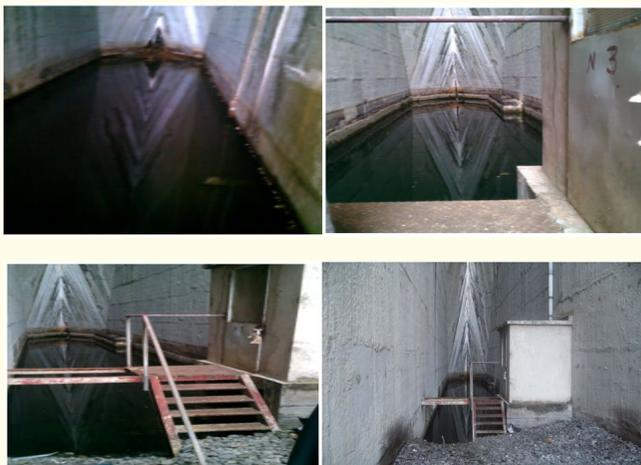
Figure 10: Figure 10 shows views of 4 plots of Shongo dam with stagnant water on the plot foot.
