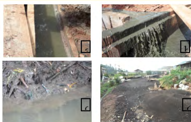
Figure 4: Direct discharge of slurry into nature (a- Nature; b- Gutters; c- Water; d- Bare Soil).
