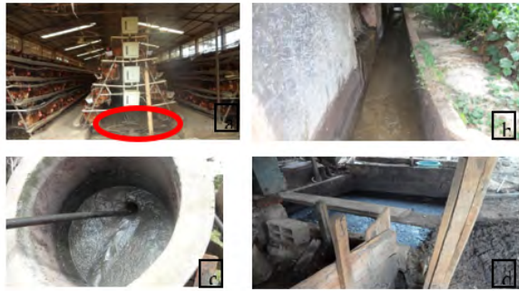
Figure 2: Collection and treatment systems for the farm's hen droppings (a: Scraper under cages; b: Collection gutter; c: Digester feed tank; d: Digestate collection pit).
