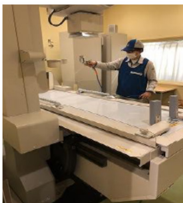
Figure 2a: Coating work in the locker room with Health Bright®. Figure 2b: Coating work in the X-ray room with Health Bright®. Figure 2c: Coating work in the blood collection room with Health Bright®.
