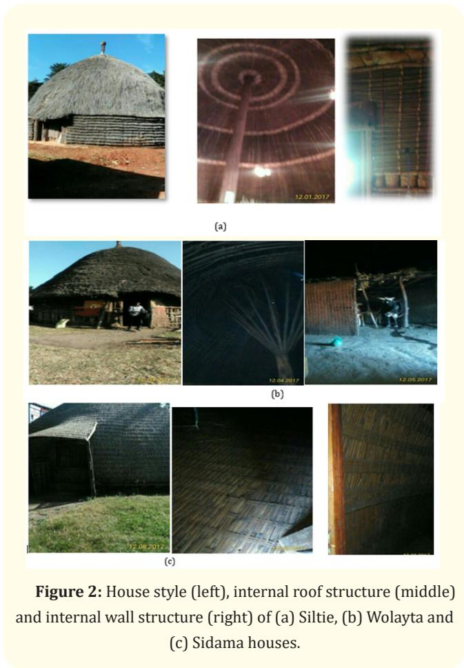
**Figure 2:** House style (left), internal roof structure (middle) and internal wall structure (right) of (a) Siltie, (b) Wolayta and (c) Sidama houses.
