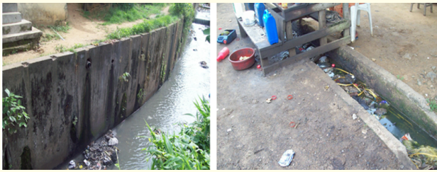
Figure 3a: Main Drainage Conduit at Bali. (Note pipe with household waste draining in to conduit).
