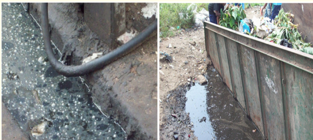
Figure 3c: Oil spills from a garage at Bali. (Note oil film in the drain)
