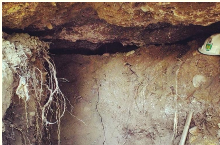
Figure 7: Entrance zone of a rubble-filled passage in the Ravne 3 tunnel, located between solid conglomerate ceiling and marlstone floor. The image captures a transitional interface at the Ravne 3 tunnel entrance, where the ceiling is composed of lithified Ravne Conglomerate, the floor consists of Miocene marl, and the side walls contain loosely compacted, unconsolidated fill material. This composition is consistent with other observed segments deeper in the tunnel system and highlights the layered and intentionally sealed nature of the passage. Root systems intruding from above and the partial exposure of geological boundaries provide visual confirmation of distinct strata.
