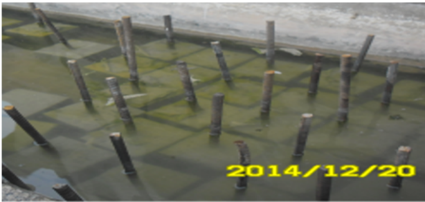
Figure 5: Curing of specimen.
