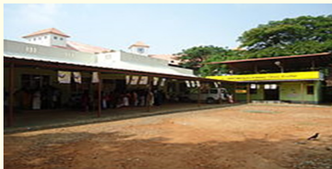
Figure 1: A community health centre in Kerala.
