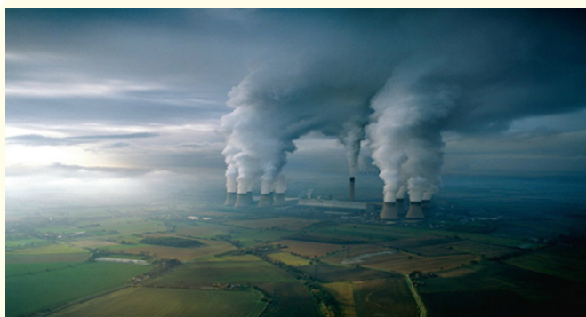
Figure 2: Shows a photo of the cooling tower: https://acs-nnov.ru/gradirni-tec.html .
