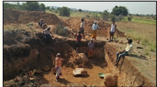
Figure b: Construction of Farm Pond
