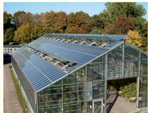
Figure 2: Solar Panel on Greenhouse. Source: http://bmrnews.com
