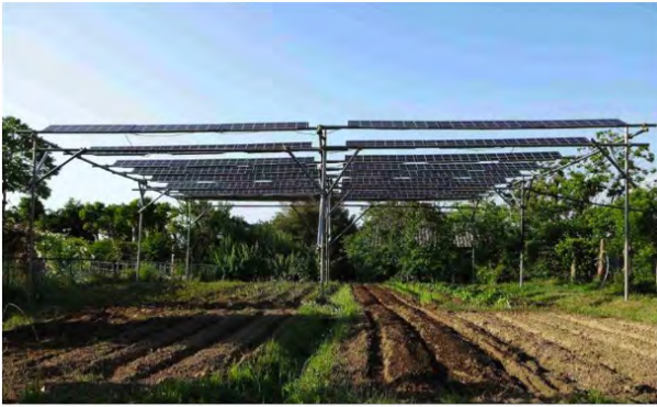
Figure 1: Solar plant with elevated structure over farm land. Source: https://www.renewableenergyworld.com
