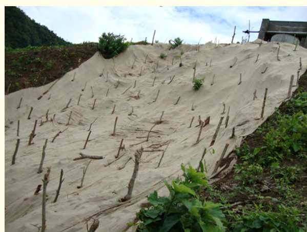
Figure 4: Reclamation of degraded sloping land by Geojute, Photo Credit: A. M. Zahid, SRDI.
