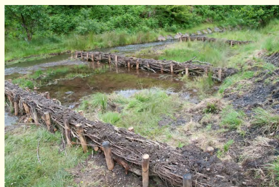
Figure 9: Brushwood check dams.
