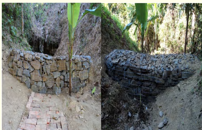
Figure 6: Gabion Check Dam (Front View at the left & Back View at right with Apron), Photo Credit: A. M. Zahid, SRDI.
